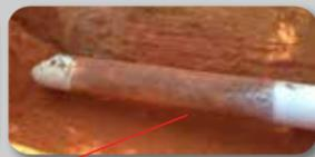
The undercutter cuts a smooth flat surface for ease of access for maintenance under and around the pipe
