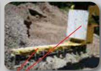
The undercutter is lined with HDPE Plastic for increased safety preventing metal to metal contact with the pipe
